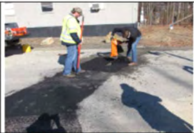
Figure 5. Bond-X spread & raked
