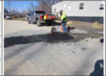
Figure 7. Both Compacted with Flat Plate
