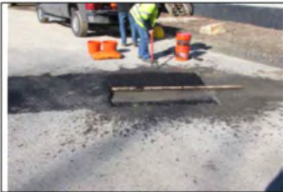
Figure 4. Aquaphalt spread & raked
