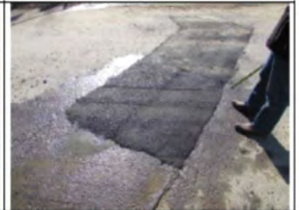
Figure 9. Loaded Tandem Axle Truck Rut
