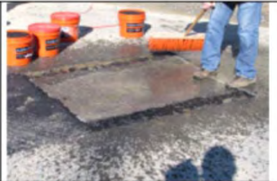
Figure 3. Area cleaned, wetted, & broomed near side Bond-X, far side Aquaphalt
